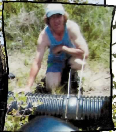
FIG. 2-B Volunteer Steve Reddy is using the right ties!
